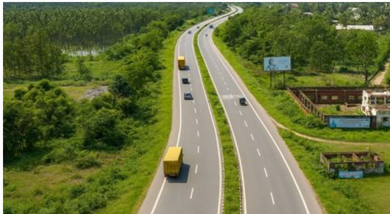
Uttar Pradesh Moradabad Bareilly Expressway Limited
